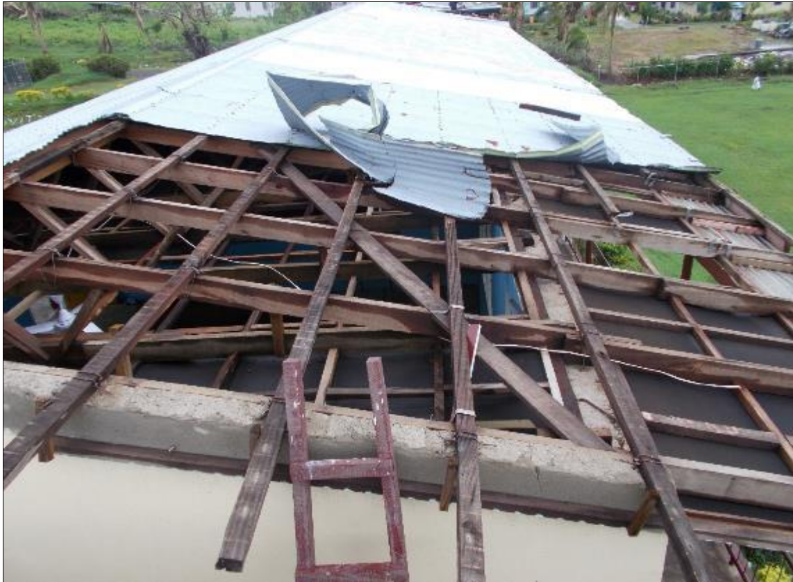
Photo 9: Showing Roof View
