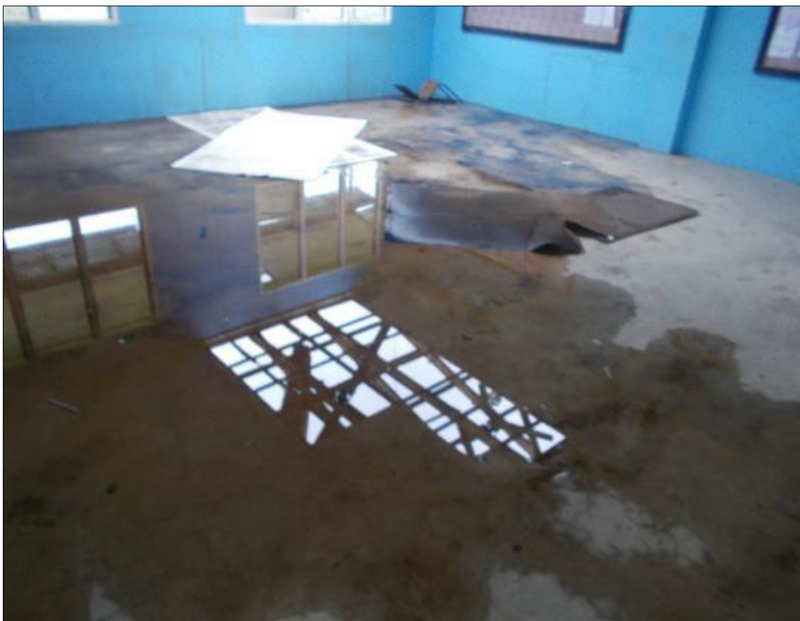
Photo 10: View of ponding floor
