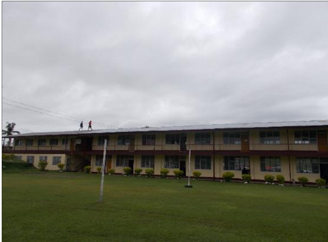
Photo 5: Front View of Block C
