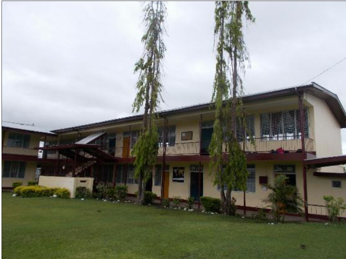
Photo 7: Side View of Block C
