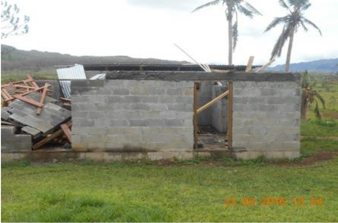
Photo 8: View of the Toilet Blocks
