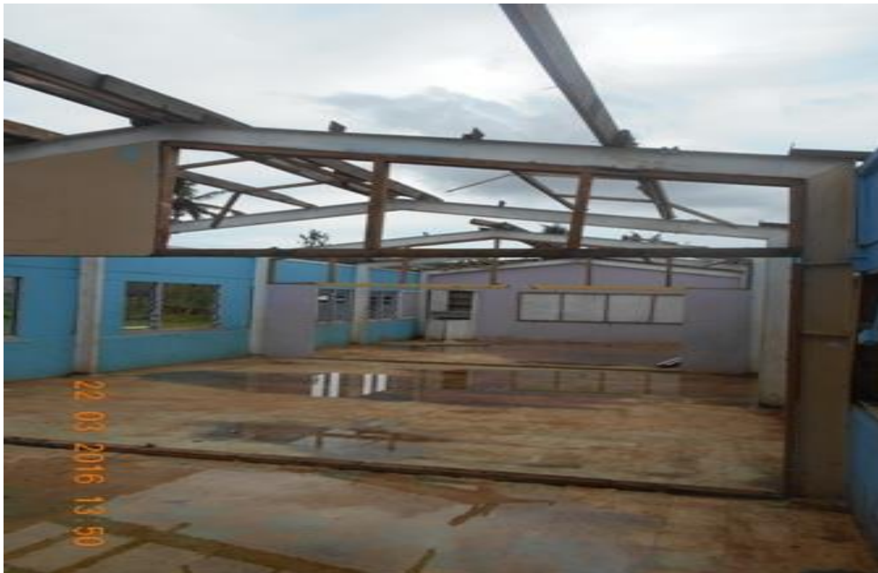
Photo 4:View of the Steel Columns and Beam in School Building
