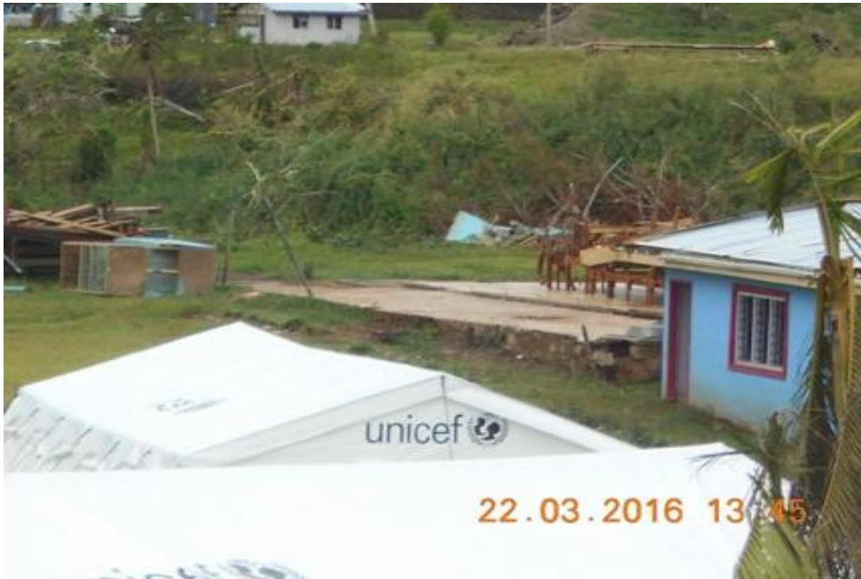
Photo 5: Overall View of Damaged Dining Hall
