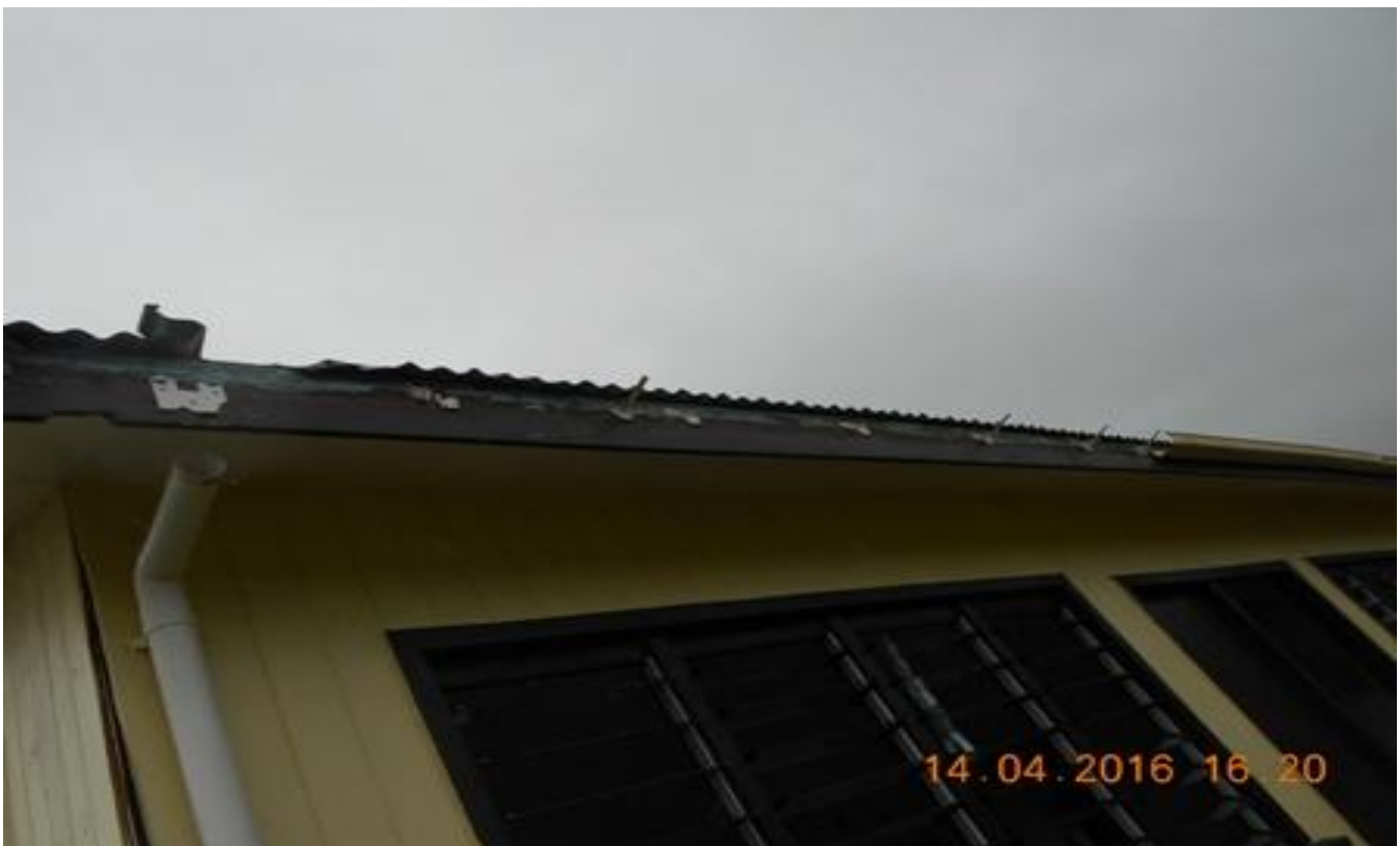
Photo 5: Damaged Gutters
