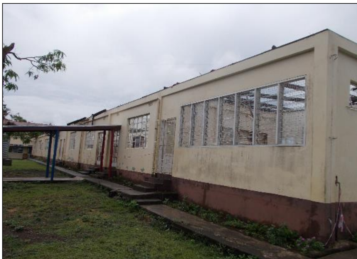
Photo 7: Overall Rear View of Block B
