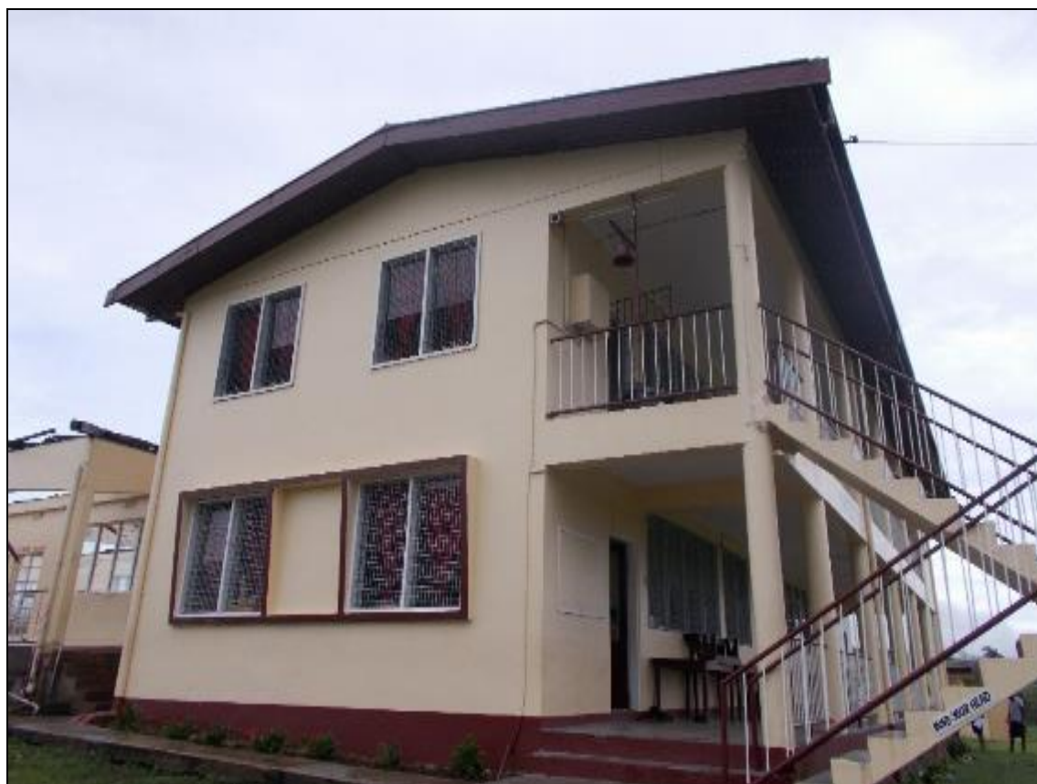
Photo 3: Gable End View
