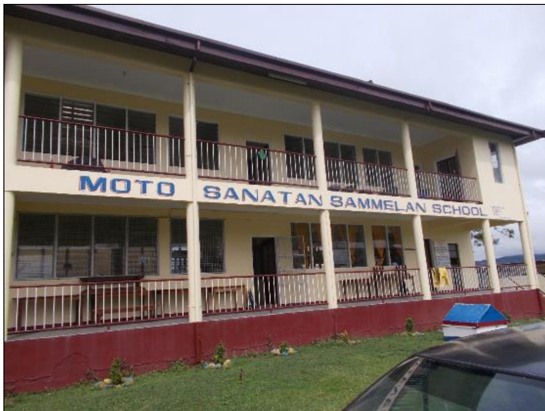
Photo 1: Overall View of Block A
