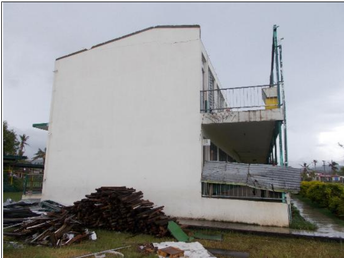
Photo 2: Gable End View of Building 1 – Block A
