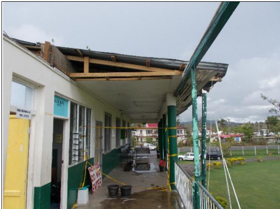
Photo 3: View of Balance of roof
