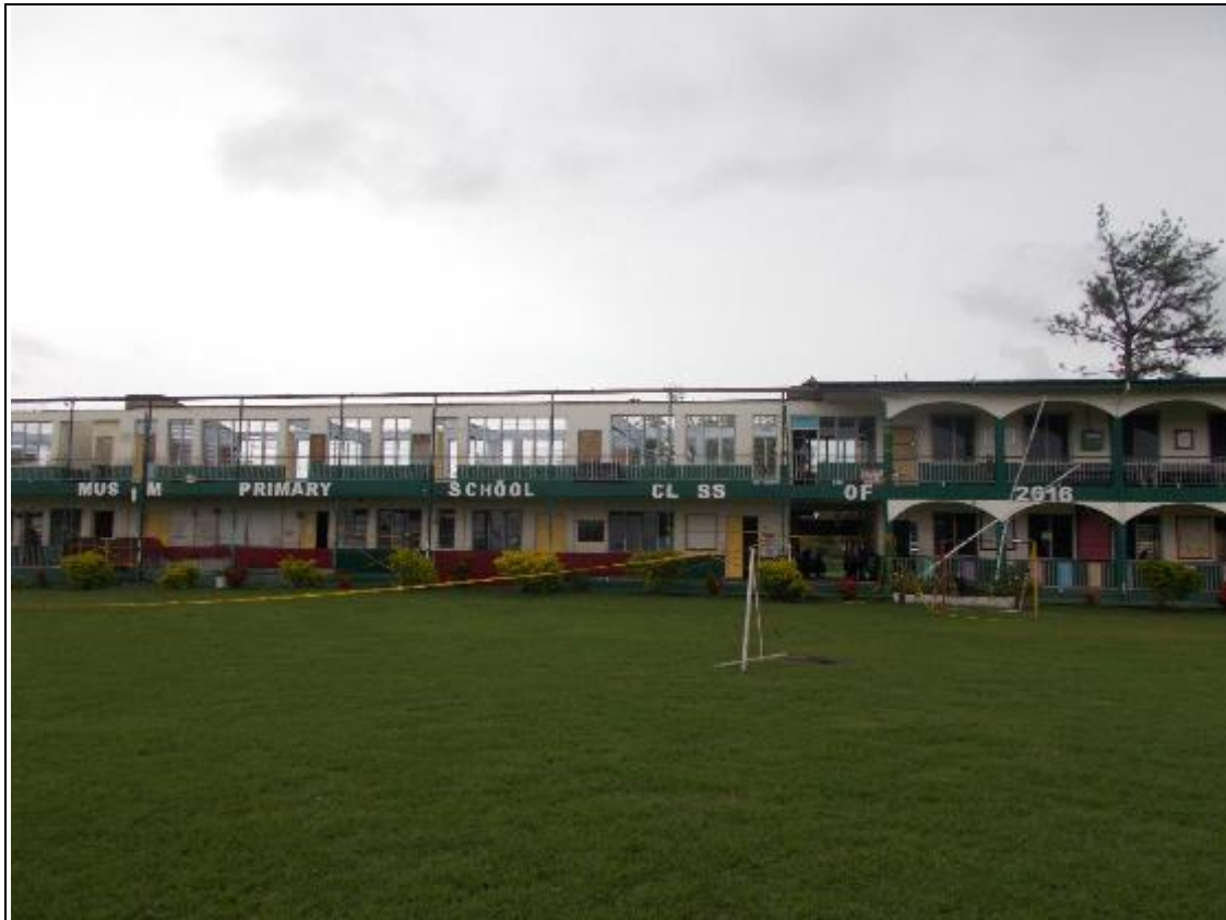
Photo 1: Overall View of Building 1 Frontage – Block A
