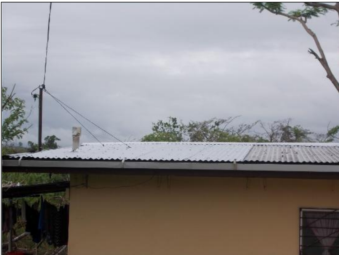
Photo 14: Showing newly replaced roof cladding
