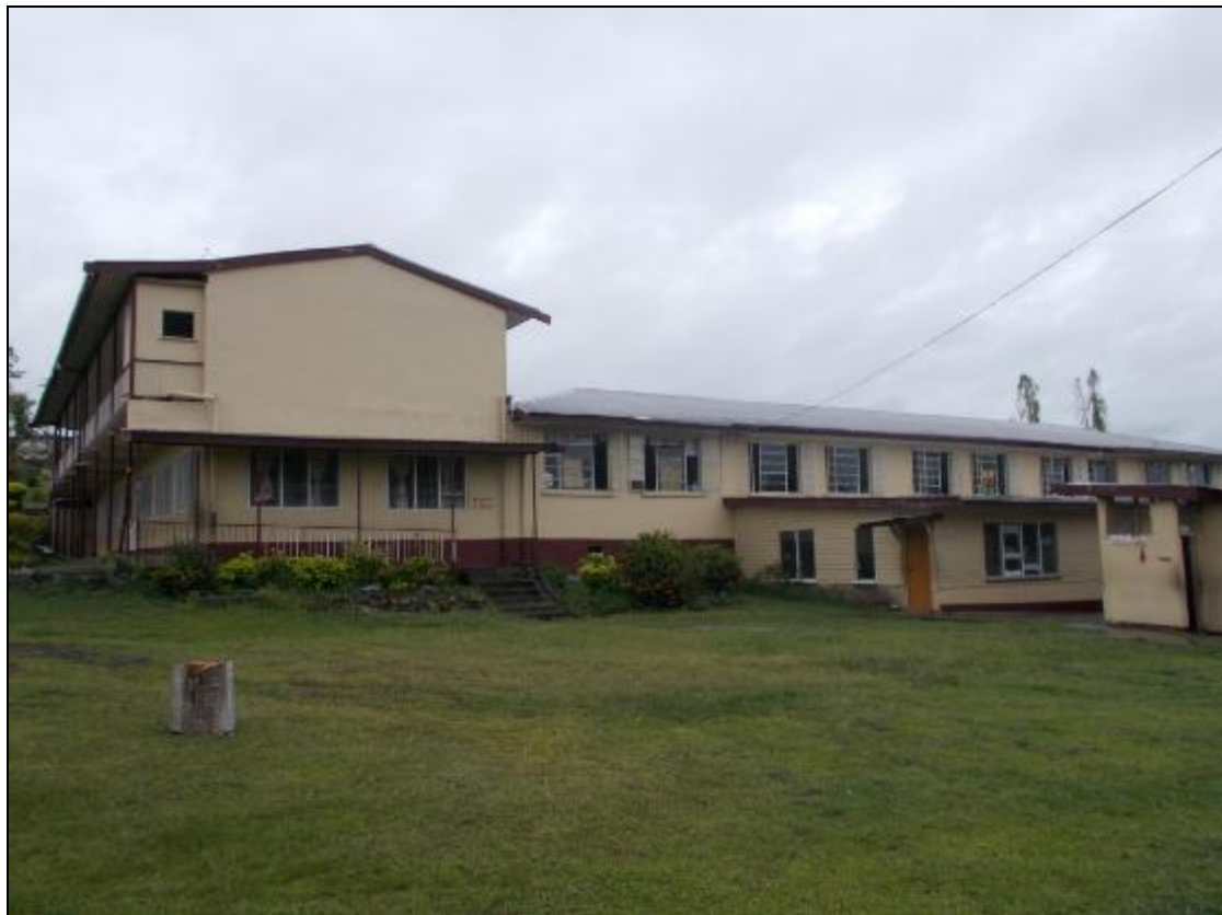
Photo 2: Overall View of Building 1 Rear /Split Level
