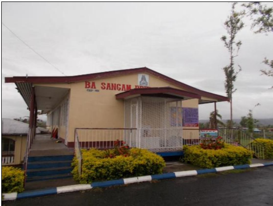
Photo 1: Overall View of Building 1 Frontage – Classroom & Admin
