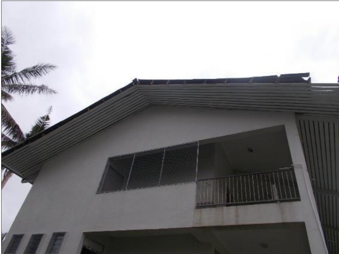
Photo 3: Side View of Building 1
