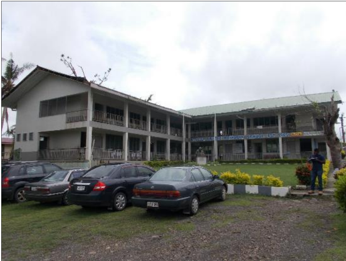
Photo 1: Overall Front View of Building 1
