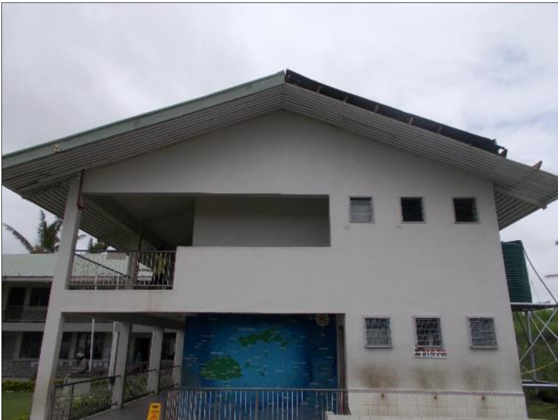
Photo 4: Side view of Building 1
