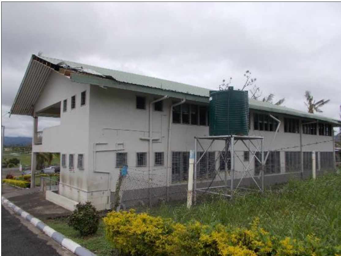
Photo 2: End View of Building 1
