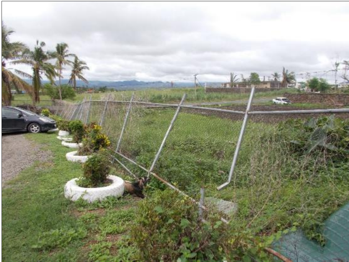
Photo 10: Showing Typical Chain-link Fence – Damaged Areas due to Fallen Tress & Debris
