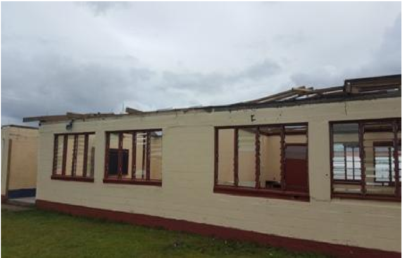
Photo 4:View of the Repairs being done at Block B
