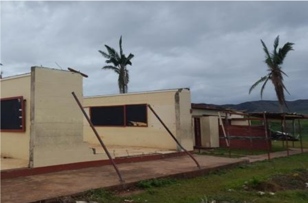
Photo 10: View of the Walkway from the Classroom to the Toilet Block
