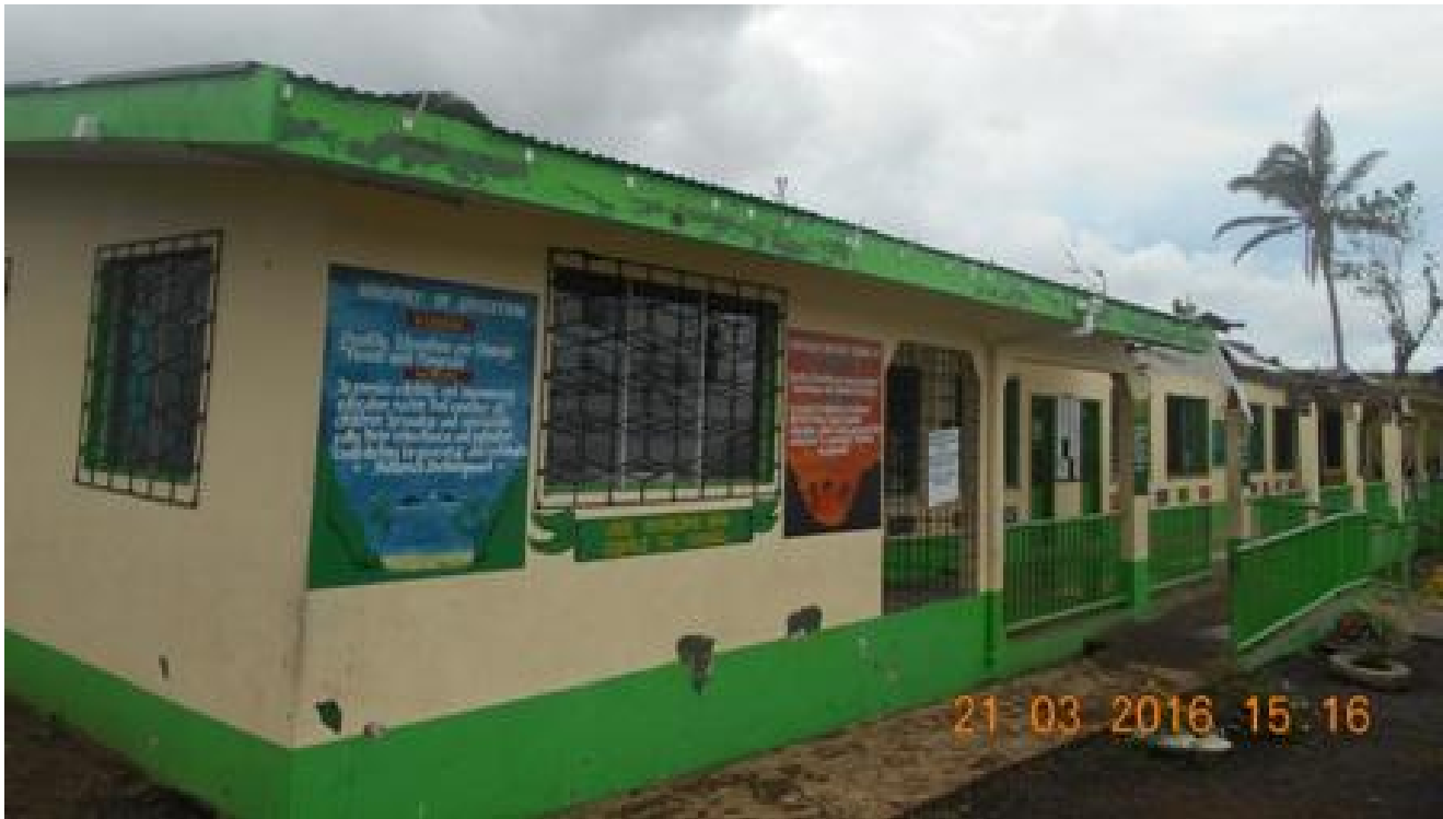
Photo 1: Overall View of Building Frontage
