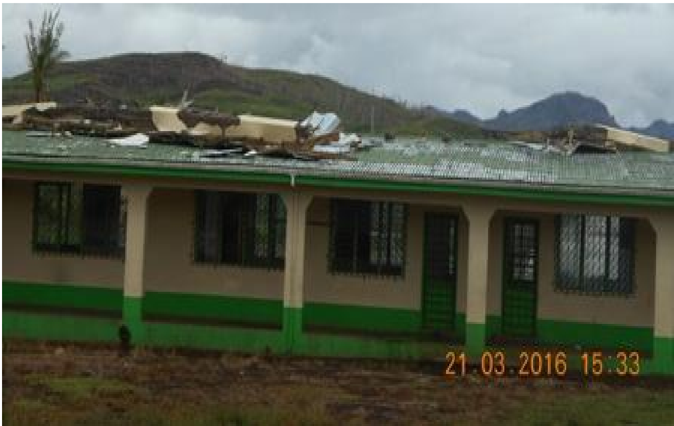
Photo 2: View of Building Rear
