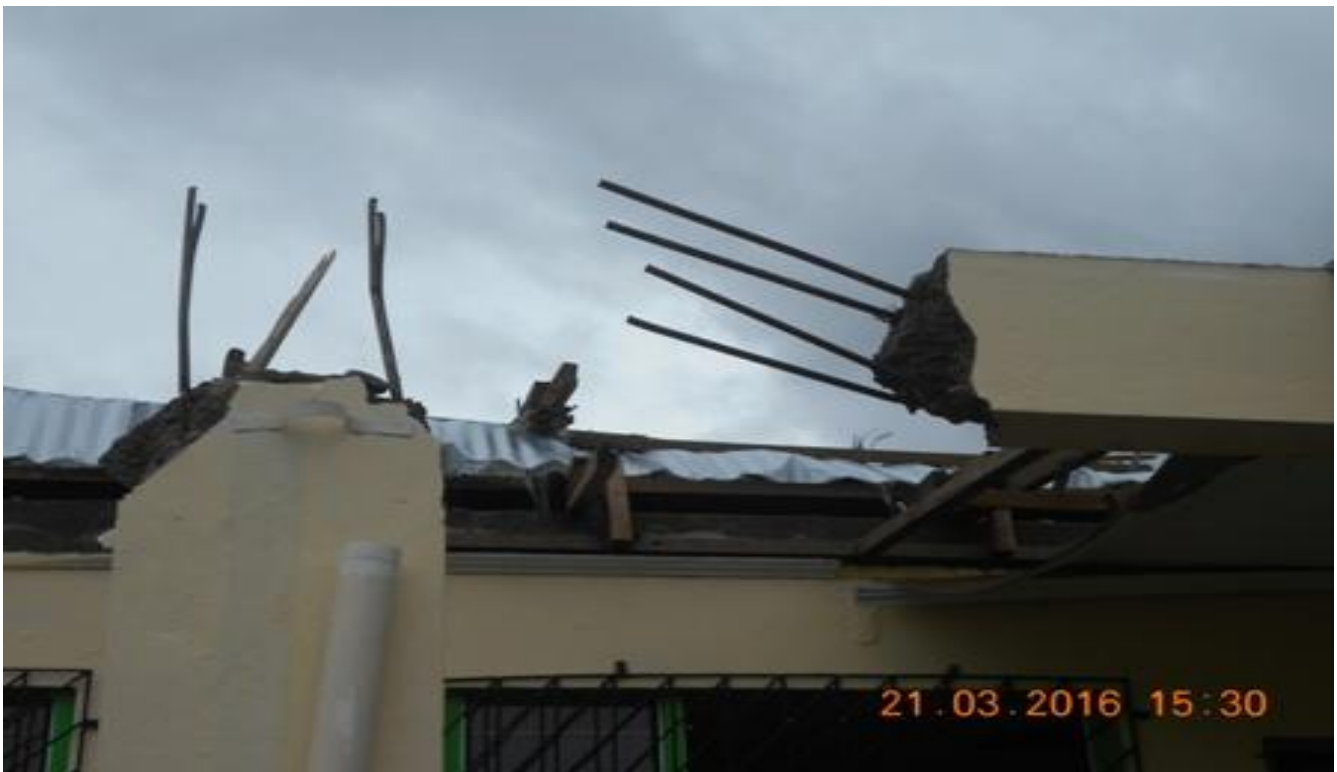
Photo 4: Beam and Column View
