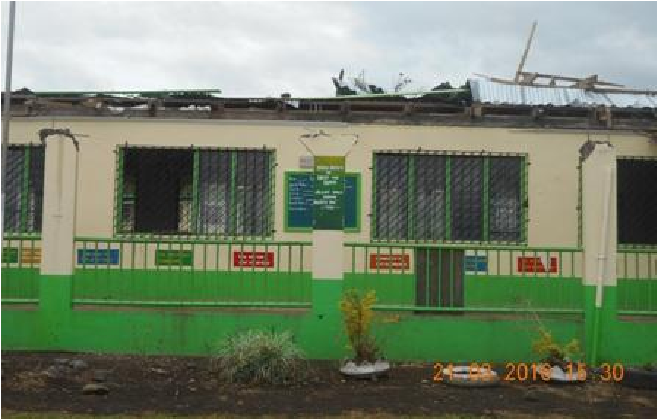
Photo 3: Verendah Beam View
