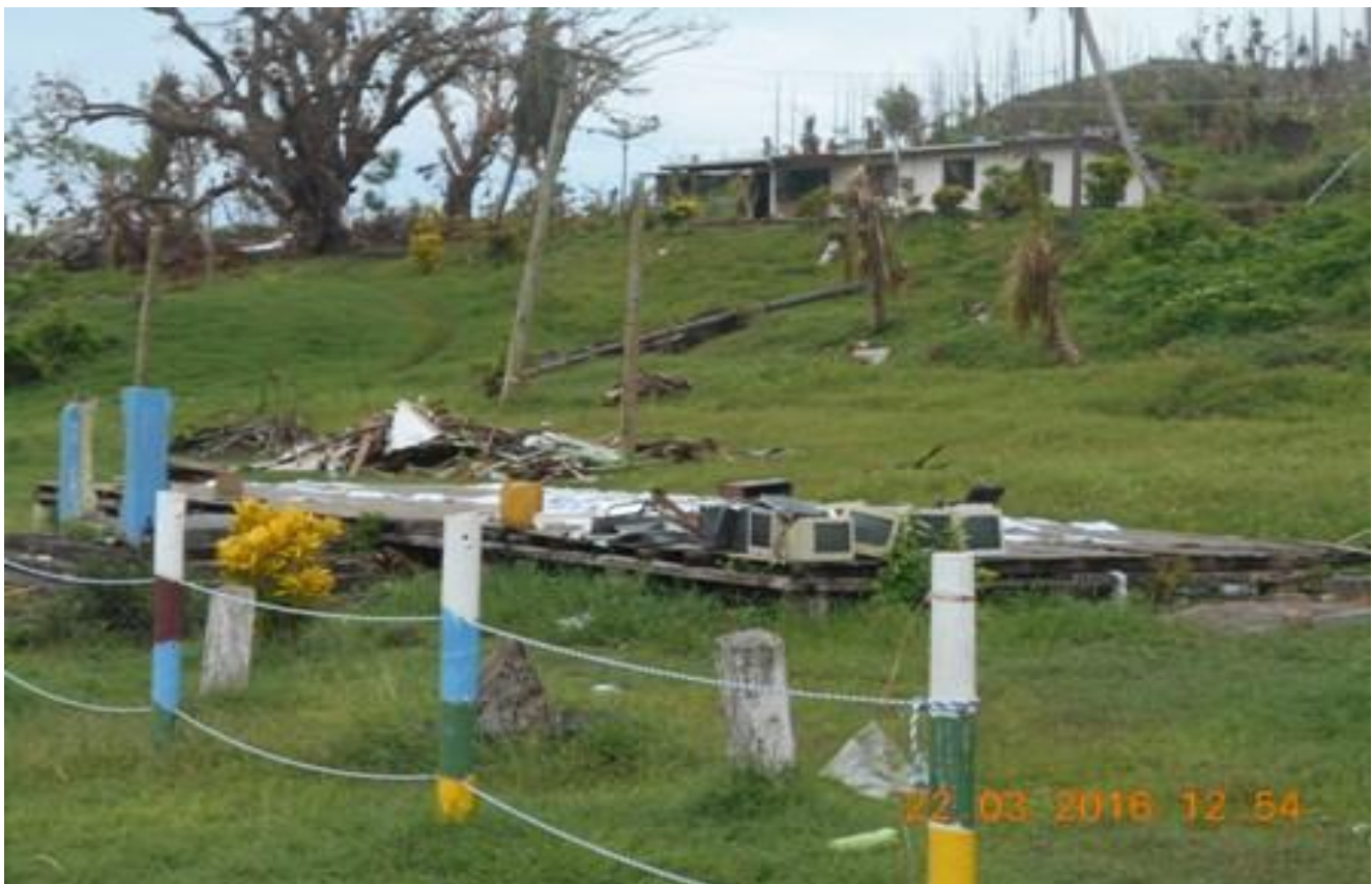
Photo 2: View of the 100% Damaged Classroom
