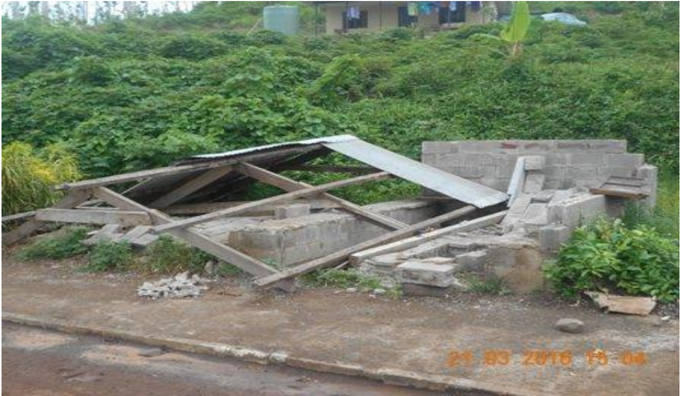
Photo 15: Showing Overall View of the Bus-Stop
