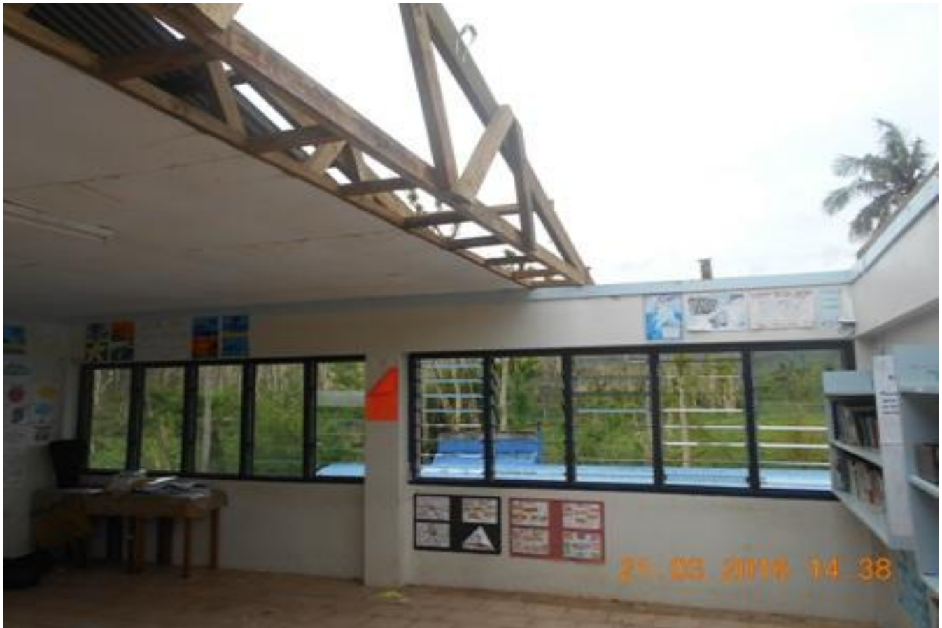
Photo 3: Truss, “U” Bolt and Louvers View
