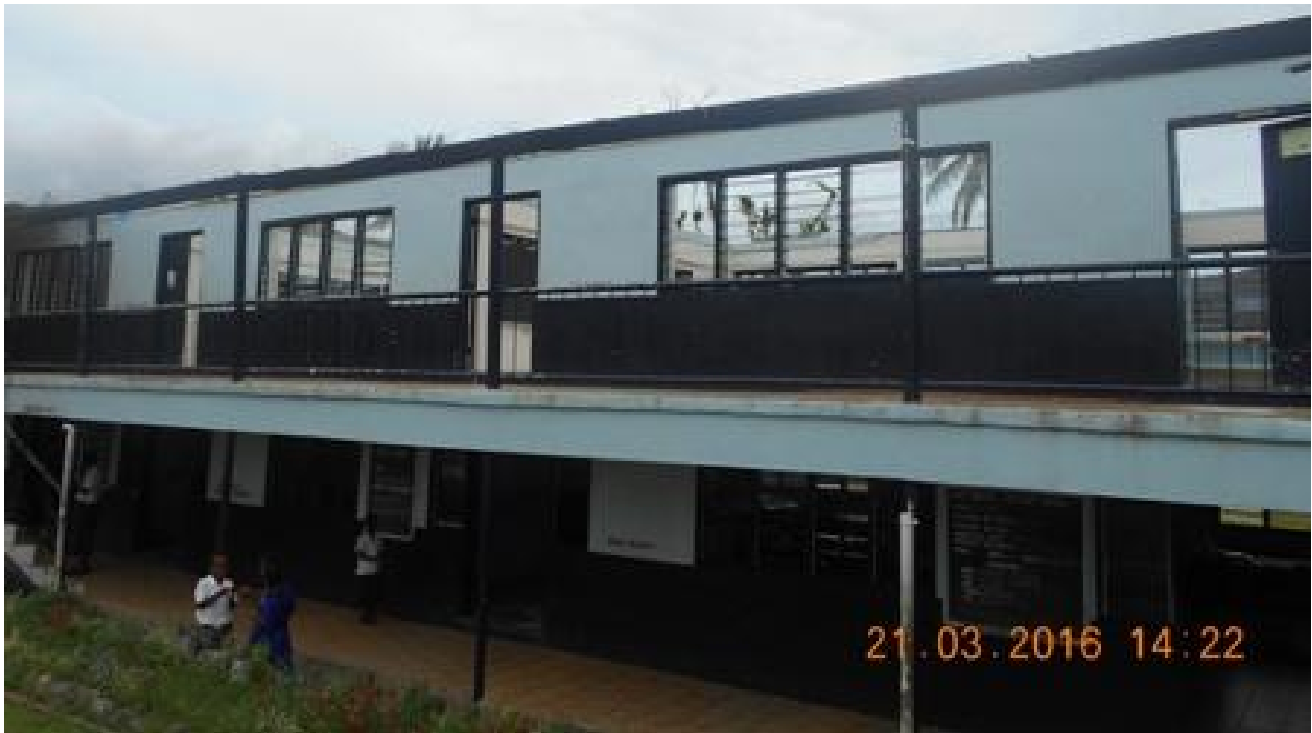
Photo 1:View of Building Frontage
