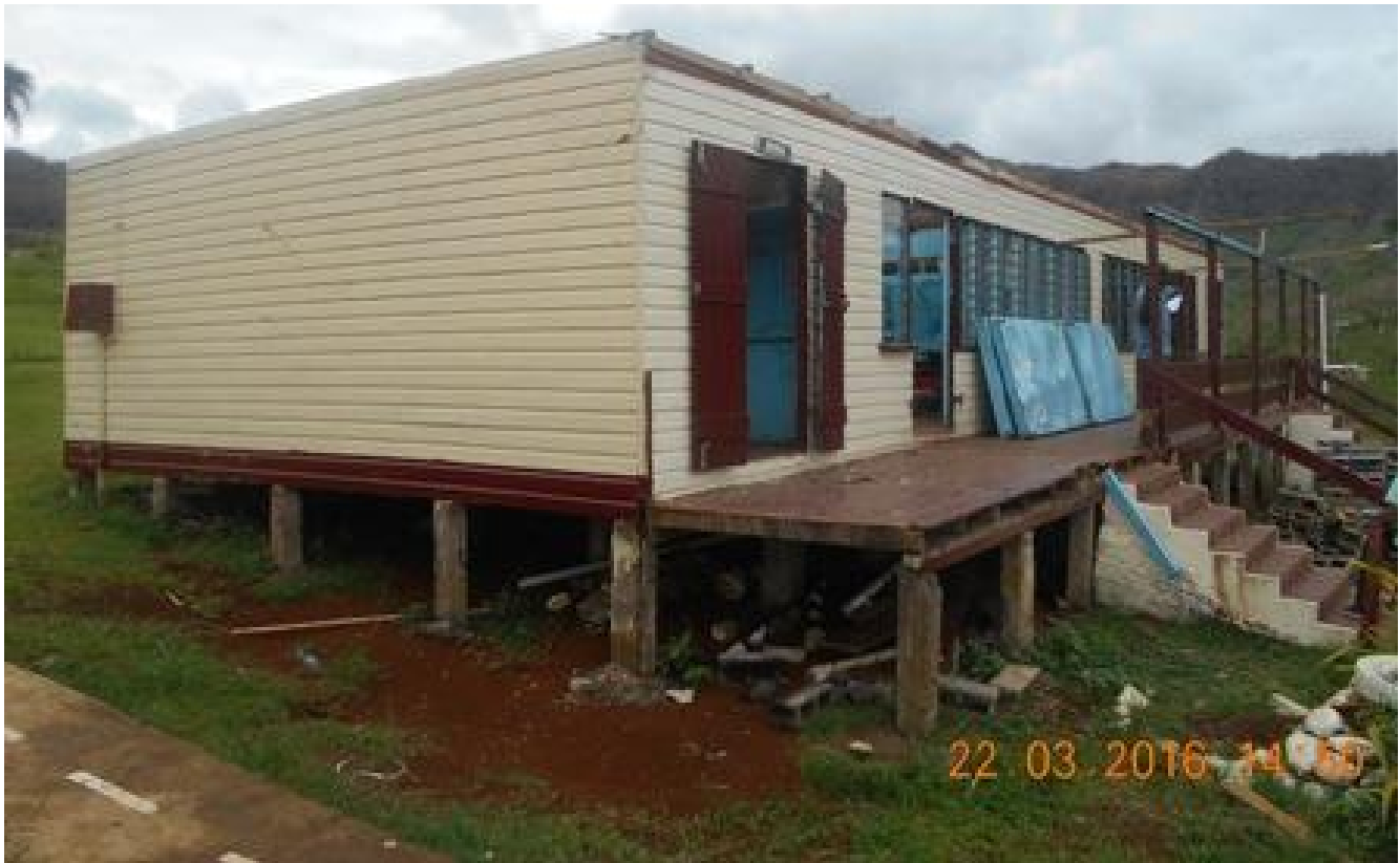
Photo 3: View of Timber Cladding Building
