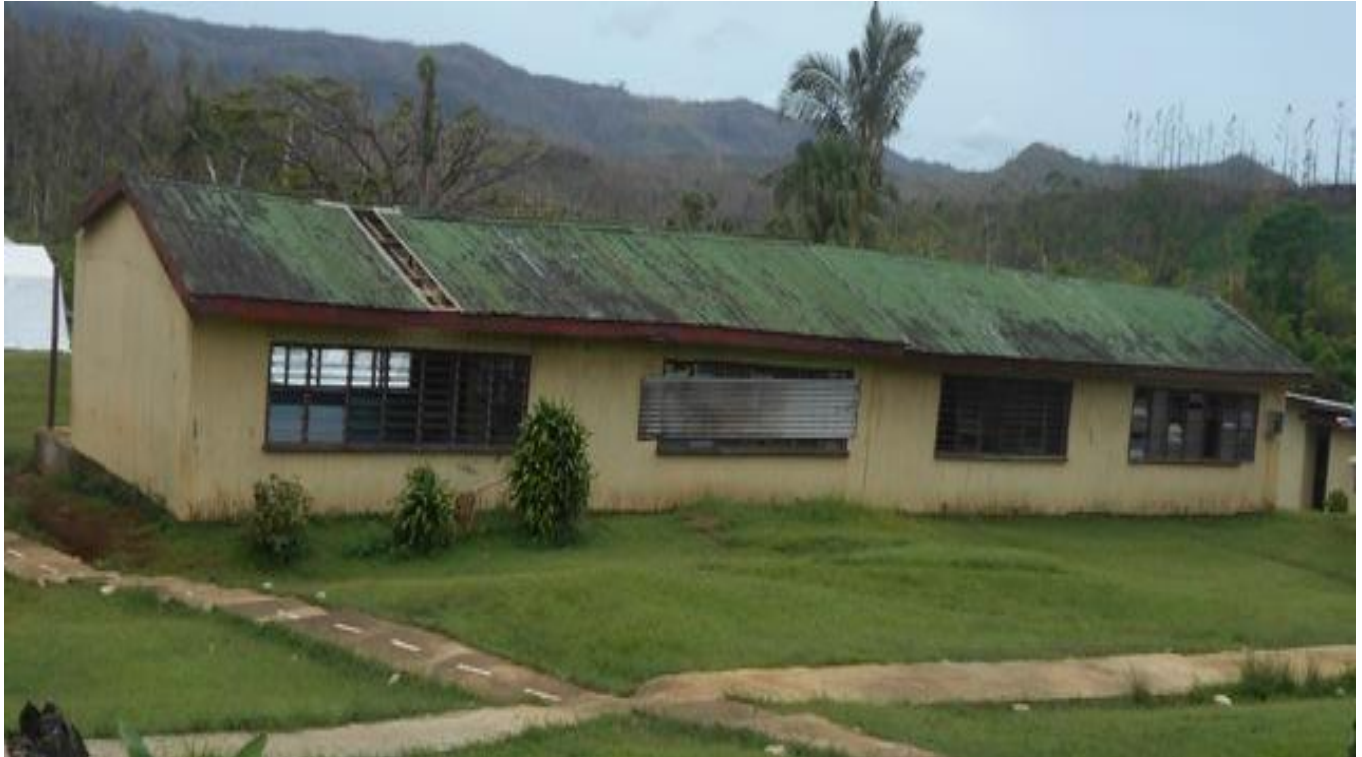
Photo 2: View of Corrugated Cladding Building
