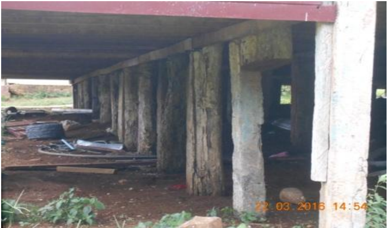
Photo 1: View of the Concrete and Timber Piles
