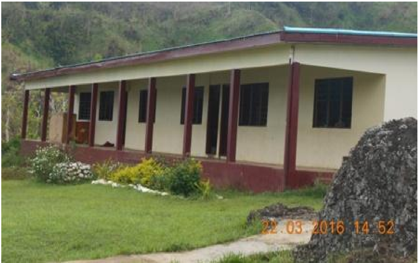
Photo 4:View of New Concrete Blockwall Building
