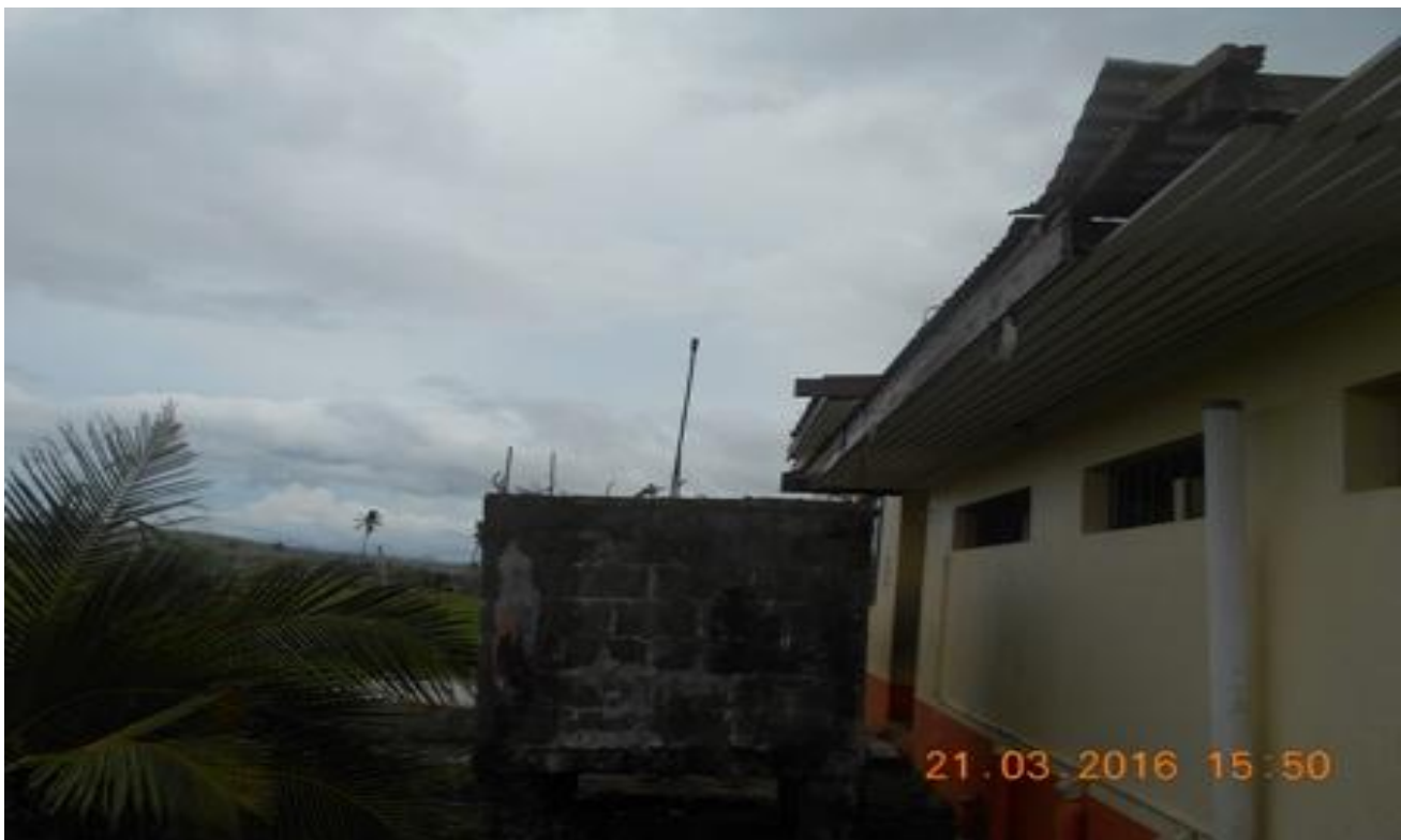
Photo 4: View of the Toilet
