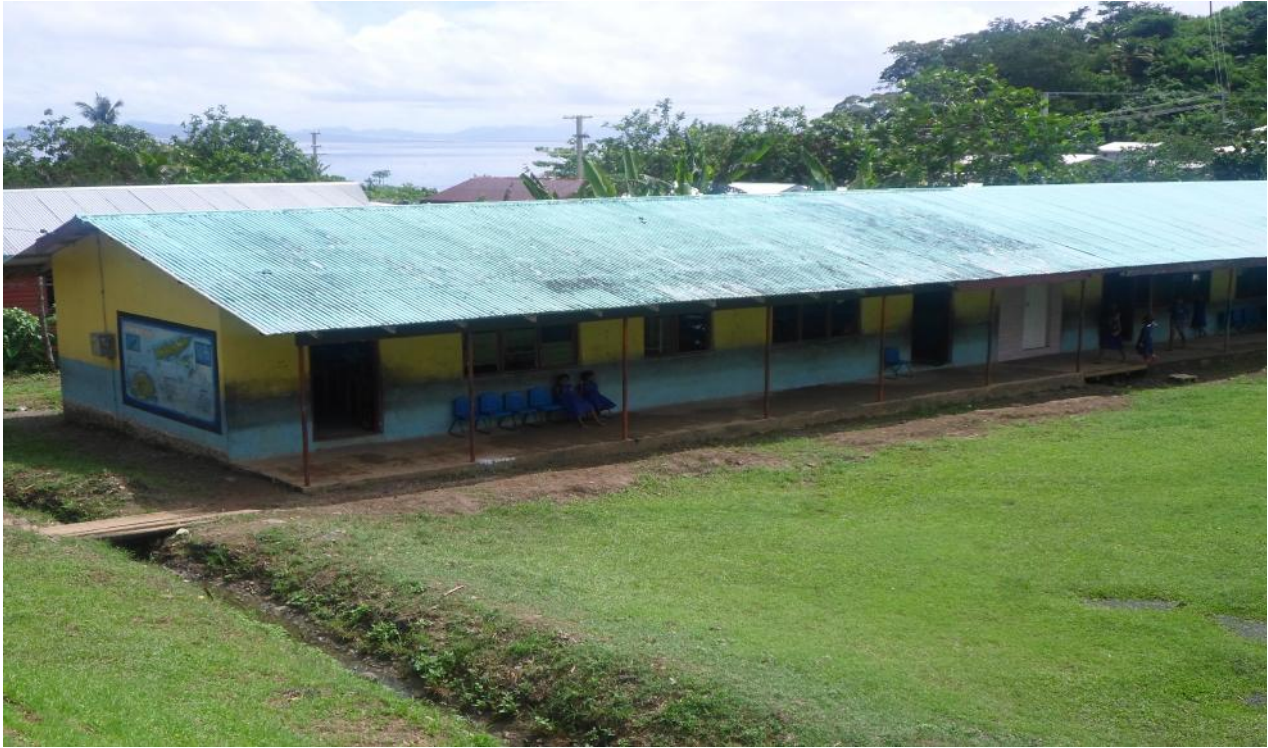
Photo 1:Rear View of Main School Block
