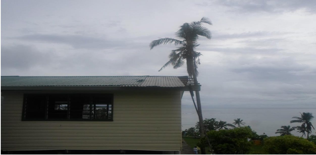
Photo 1:Rear View of Main School Block
