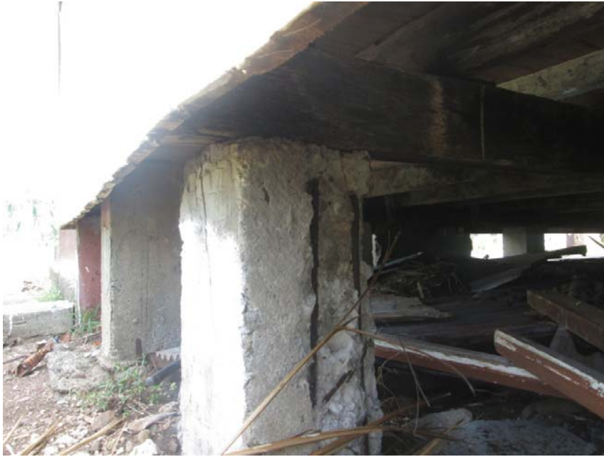
Photo 5: View of Pier
