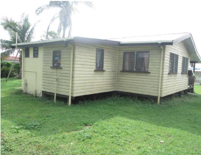
Photo 6: Side& Rear View of building 2
