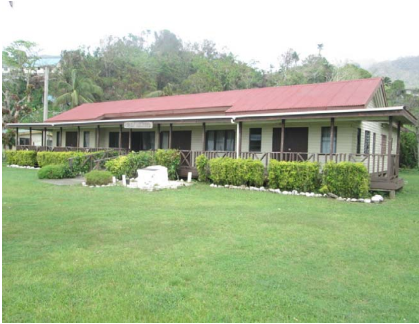
Photo 1: View of Building 1 Frontage
